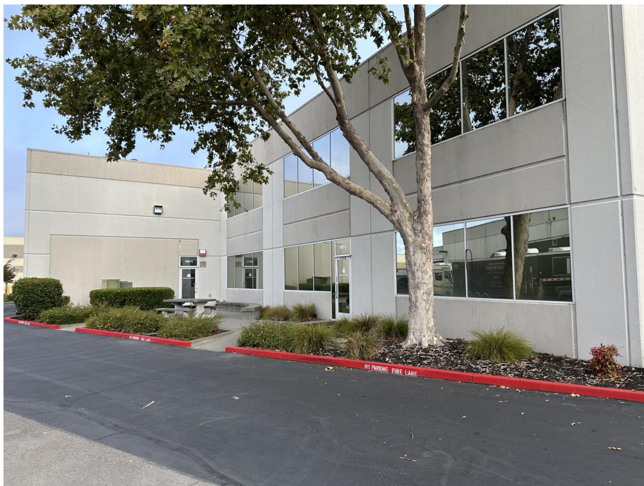
Diamond Valley, Diamond Quanta's Petaluma operations and process development center. Petaluma, California.
